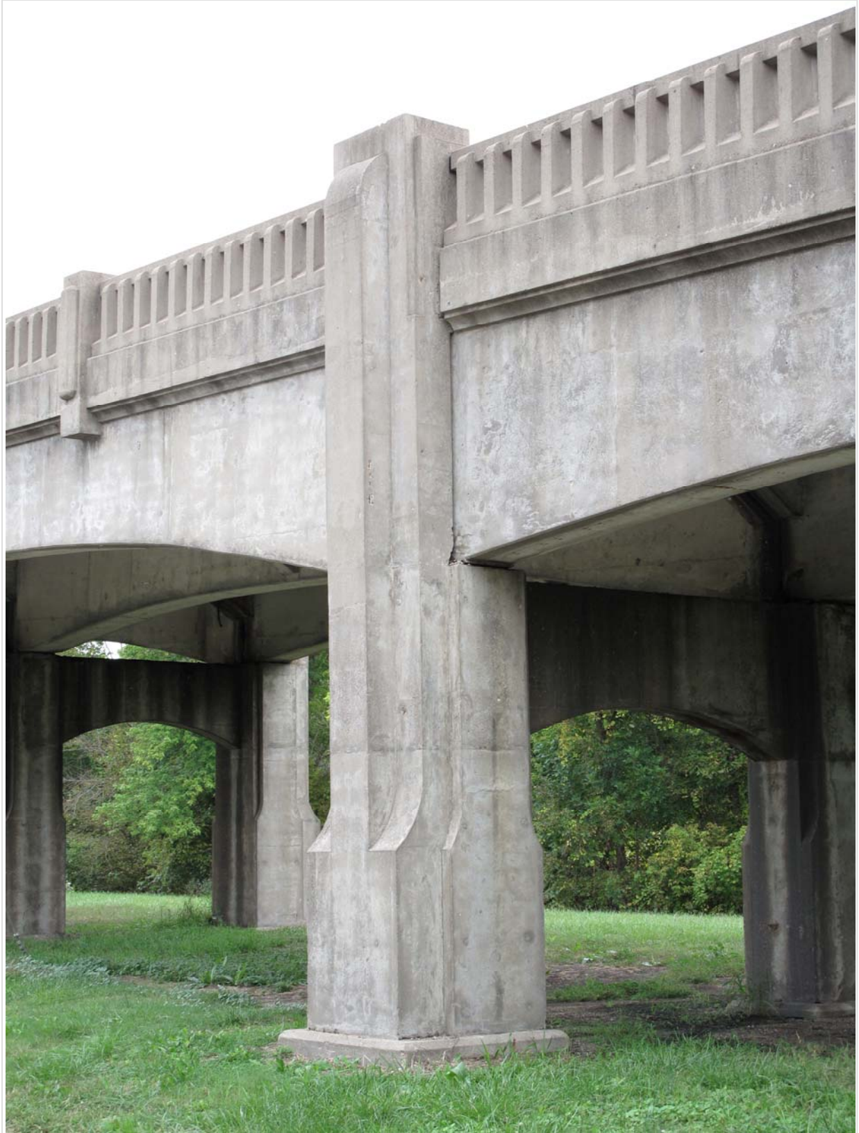
#34 of 35. Bridge K0744. Bent 19. View to northeast.
