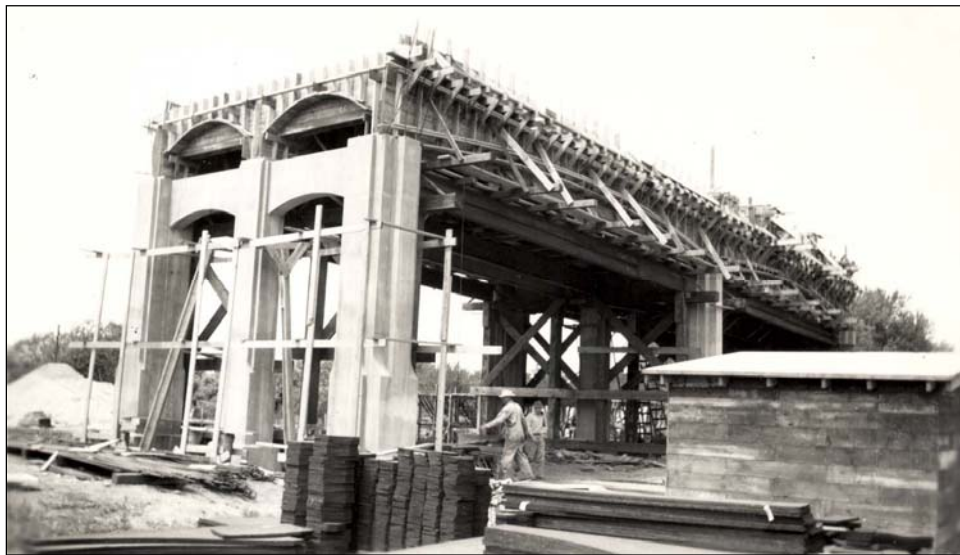
Figure 5. Forms for pouring of deck and roadway girders.
