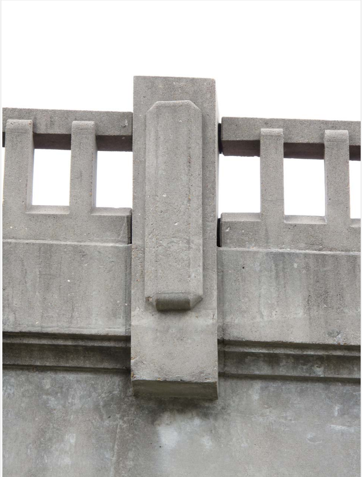
#33 of 35. Bridge K0744. Detail at Span 18-19. View to east.
