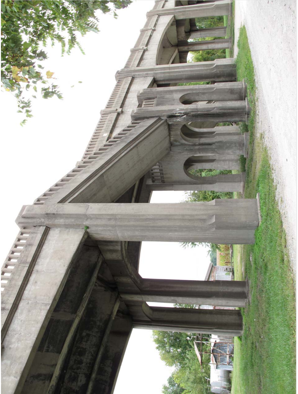
#20 of 35. Bridge K0744. Stair assembly at Span 12-13. View to southeast.
