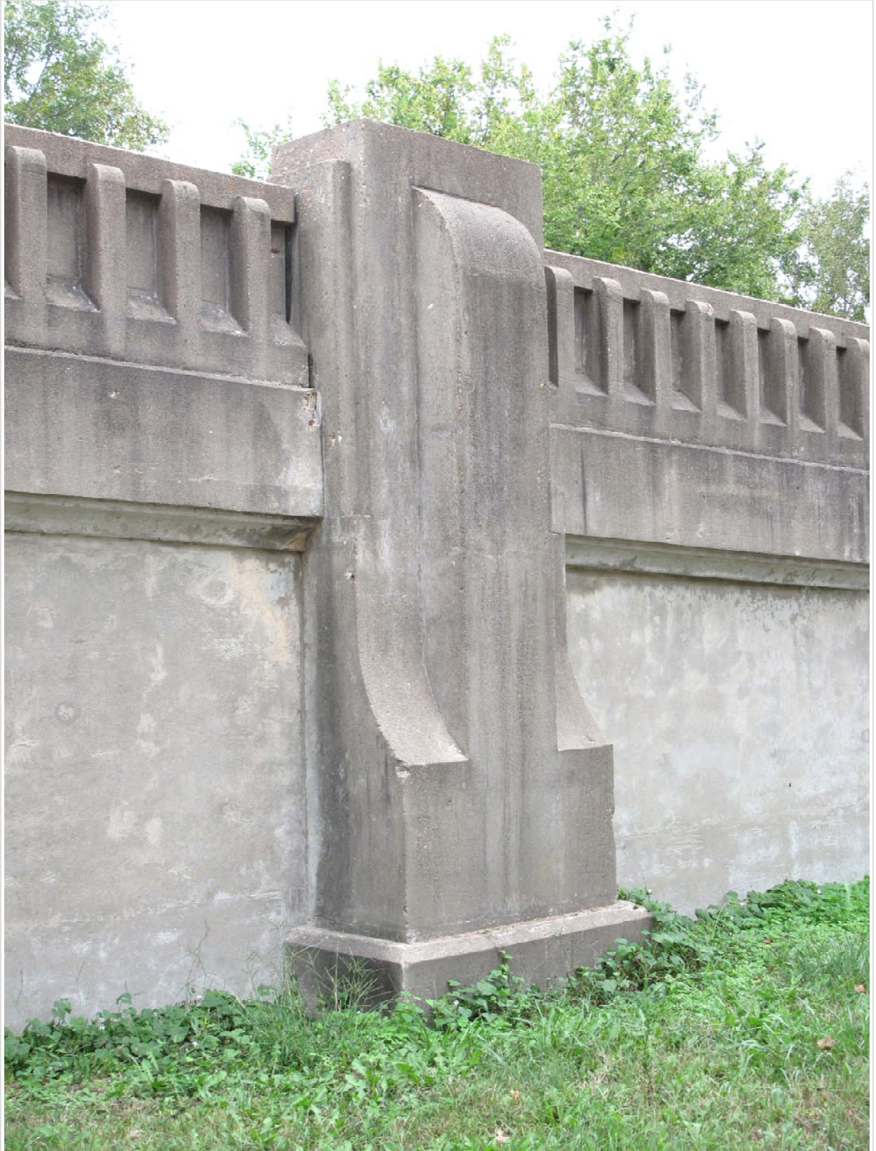
#35 of 35. Bridge K0744. Abutment 20 detail. View to southeast.
