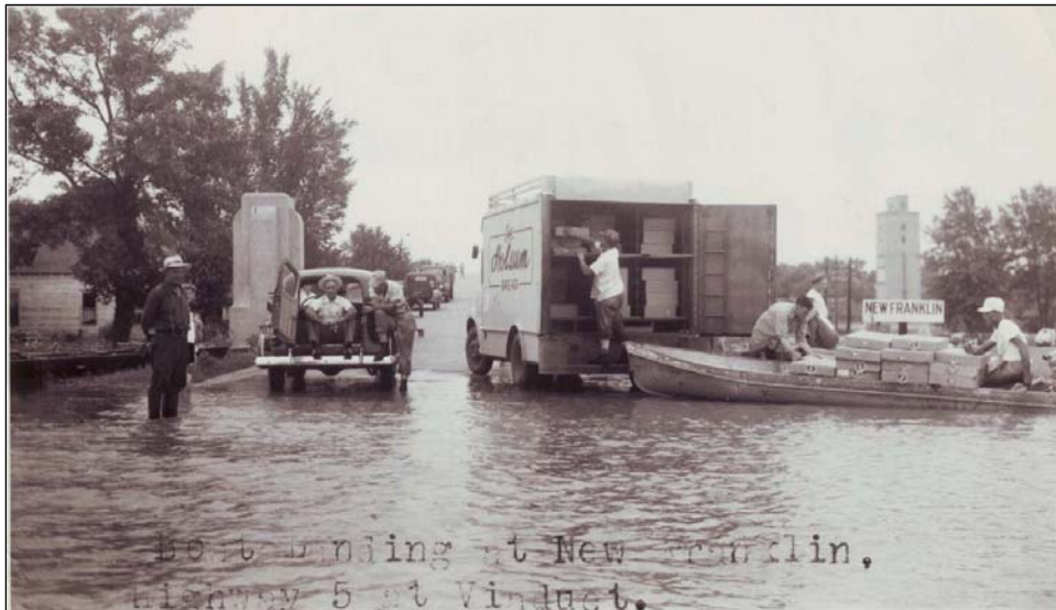
Figure 7. South end of viaduct, showing end pilaster. (Courtesy South Howard County Historical Society)
