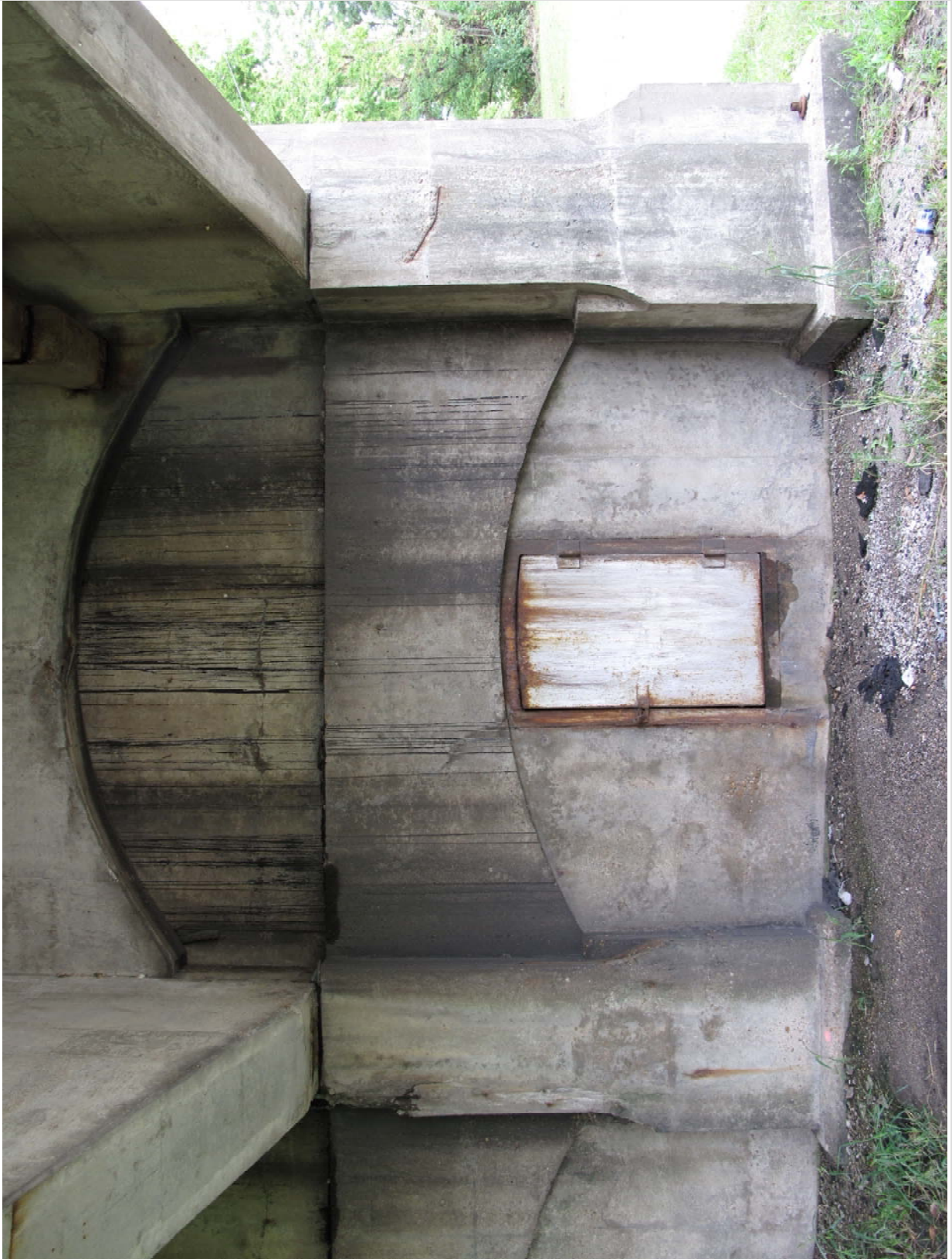
#10 of 35. Bridge K0744. Steel door at Section 1-2, Abutment 20. View to south.
