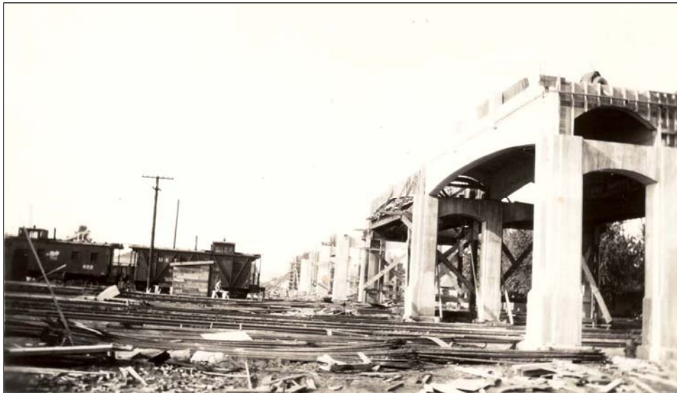
Figure 2. Viaduct construction over MKT Railroad tracks.
