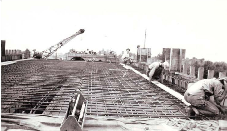
Figure 6. Reinforcing steel for roadway girder. (Courtesy South Howard County Historical Society)
