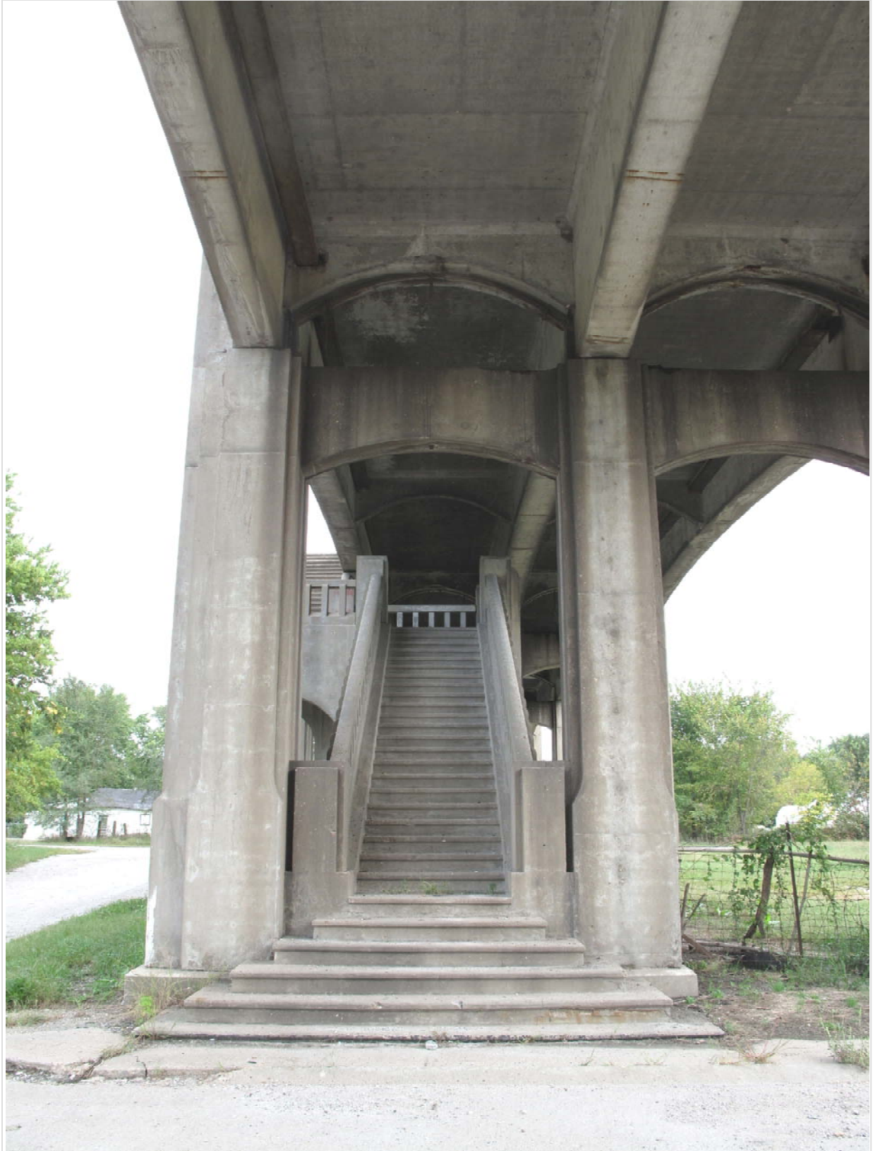
#16 of 35. Bridge K0744. Approach stairs and first run at Span 12-13. View to north.
