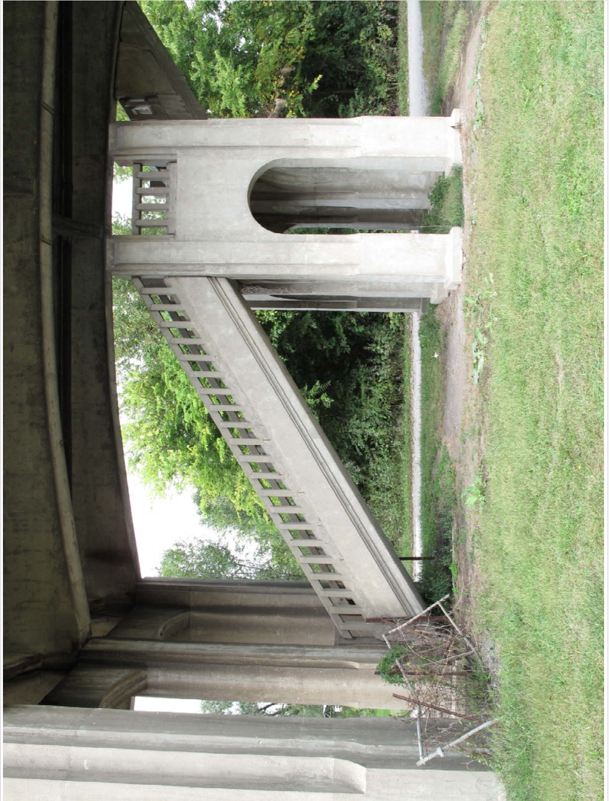
#14 of 35. Bridge K0744. Stair Tower 12A and steps at Span 12-13. View to west.
