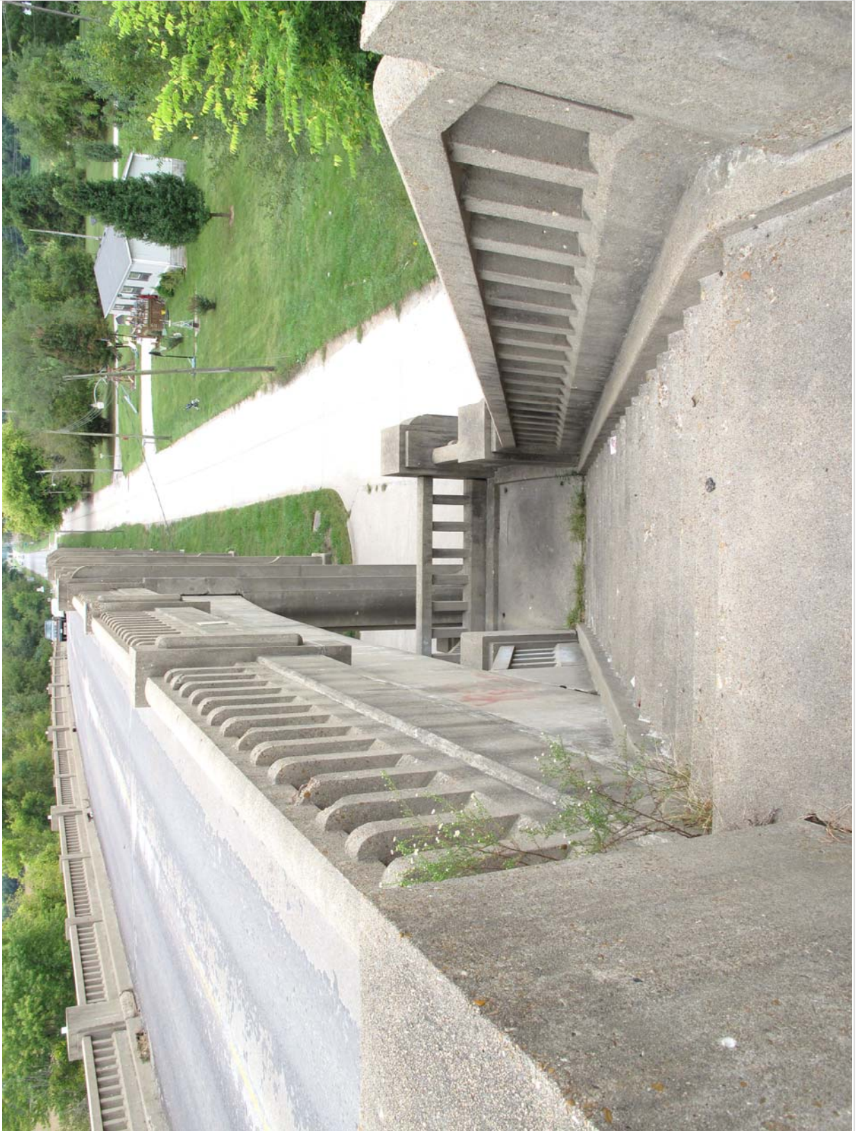
#23 of 35. Bridge K0744. Roadway, stairs, southwest side. View to south.
