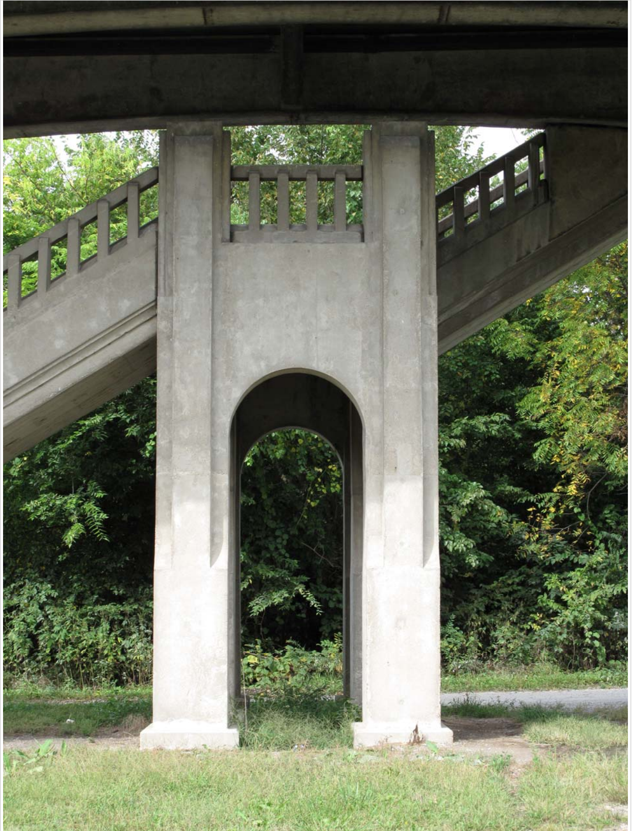
#15 of 35. Bridge K0744. Stair Tower 12A. View to west.
